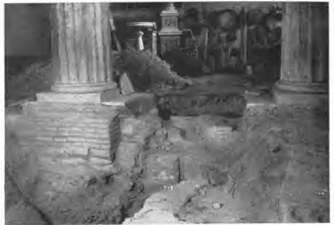
Fig. 163 a . S. Pietro in Vincoli, South colonnade, footing between columns 1, 2
